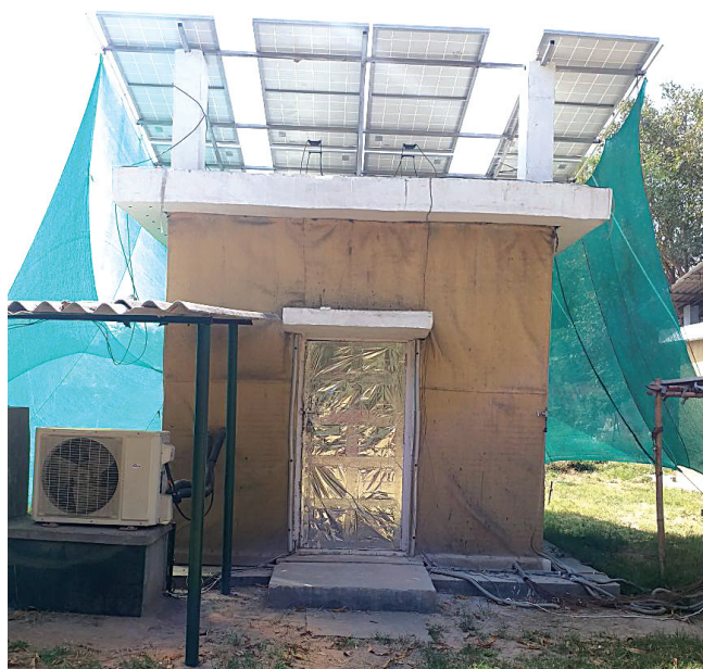
Stand-alone, batteryless, off-grid, solar-refrigerated evaporatively-cooled (SREC) structure
