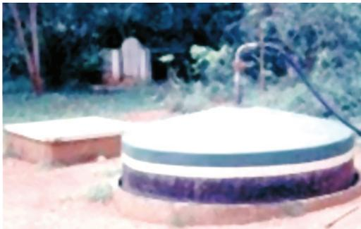
Fig. 2.1: Floating drum plant
